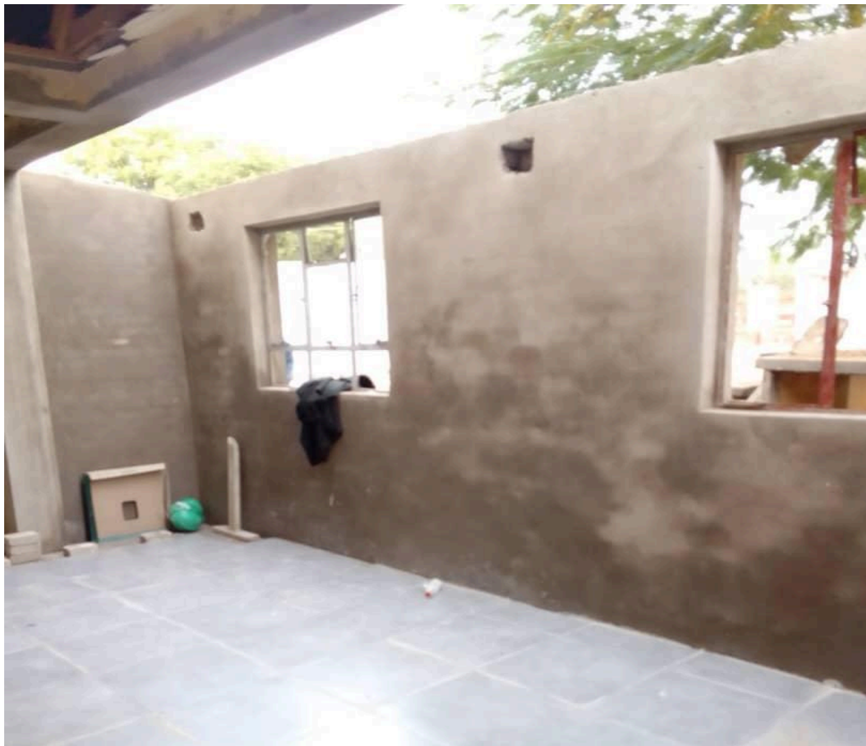
Wall being rebuilt for extension of recovery area
